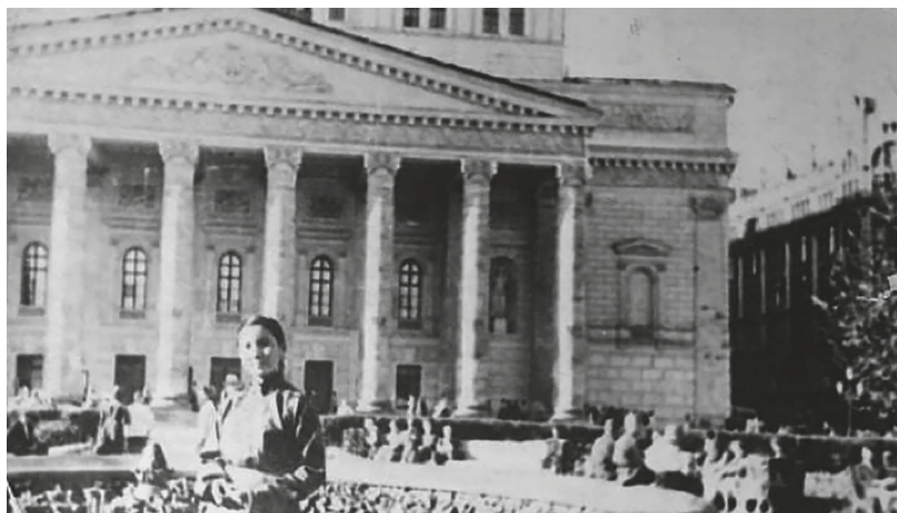
FIG 7 Ts. Khandjav standing in front of the Bolshoi Theatre in 1955. Ts. Khandjav's private collection.
